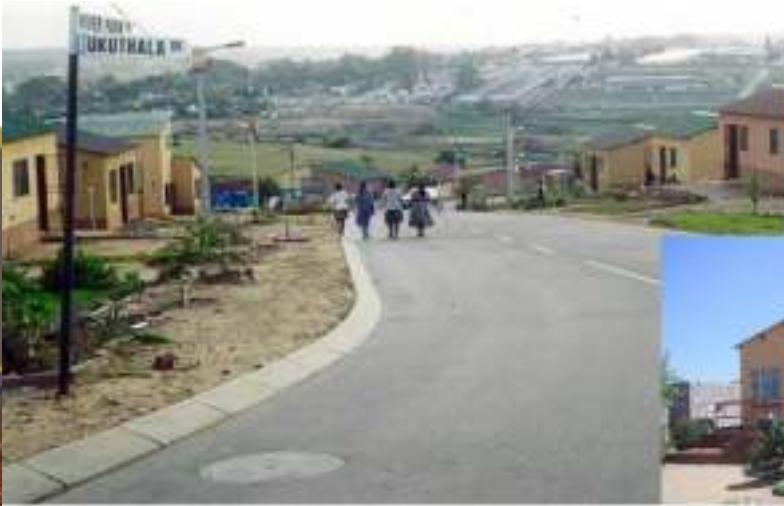
Riverpark 870 RDP houses
