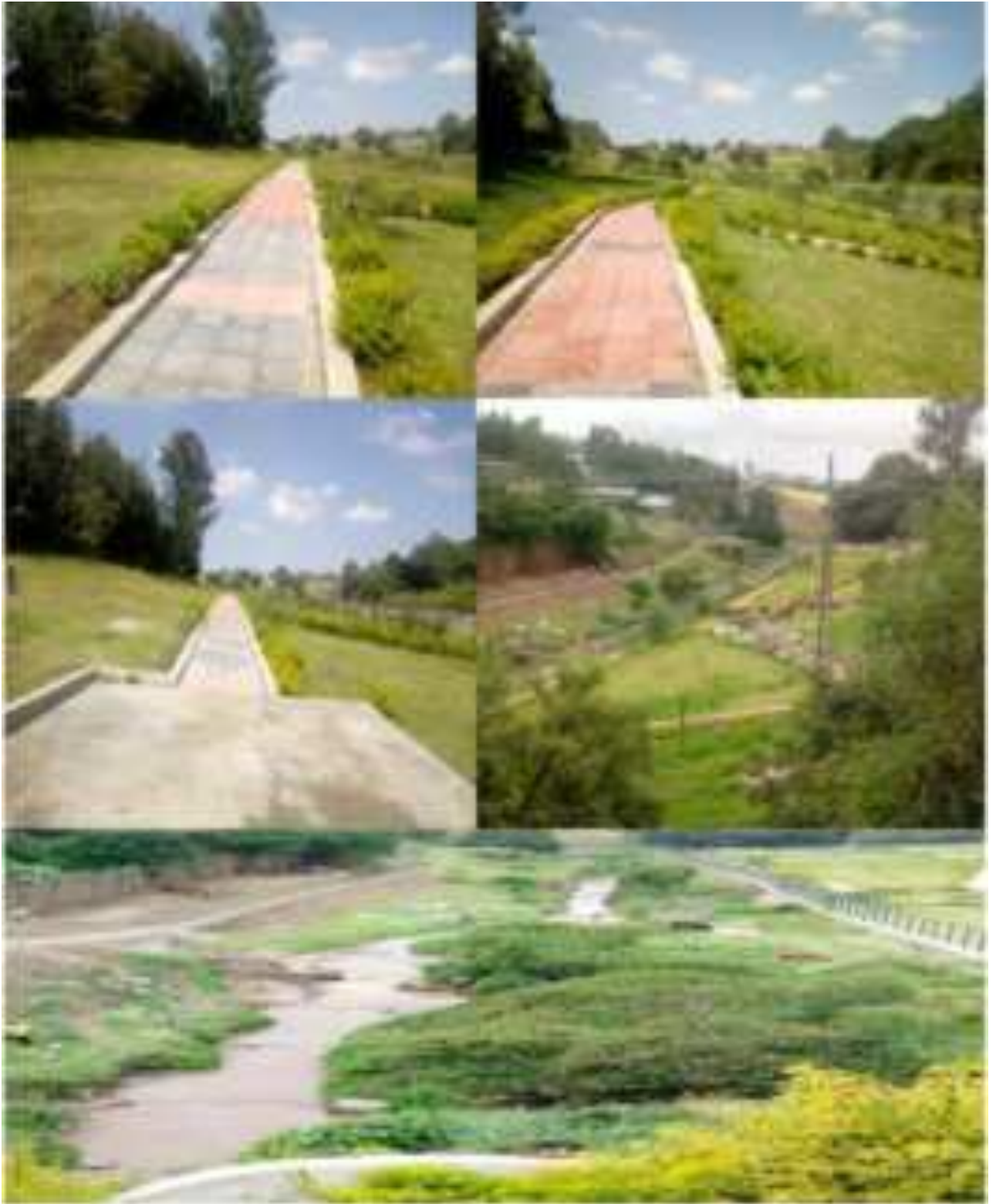
Figure 29: Hesa River Malka Kare Waterfront Development after Implementation, At Present
